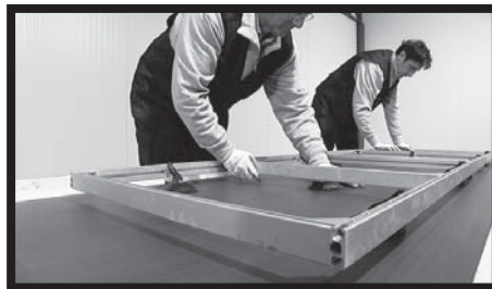
Fig.4/5 - All versions of SLIMTECH slabs, of size 300x100 cm, can be handled by two persons, using a special frame. Fix the frame to the slab when it is still on the pallet using the suction cups. Raise the frame and slab to eliminate the suction effect.
